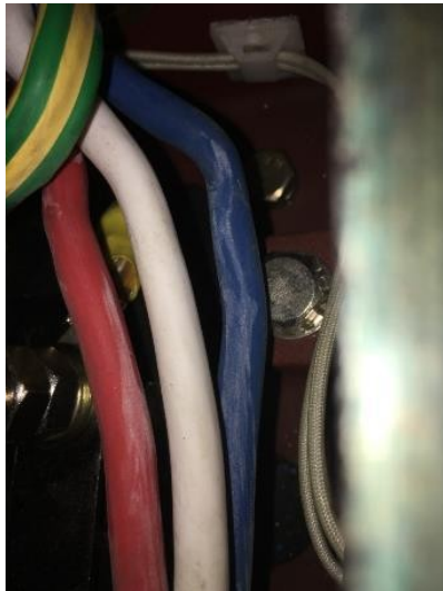
Blue Supply touching Mounting bolt
