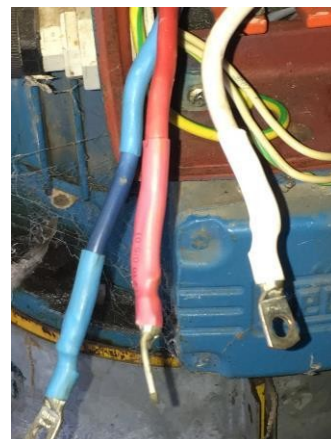
Heat Shrink repair
