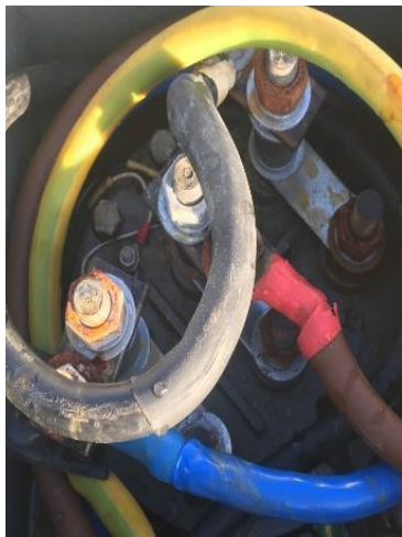
Moisture Ingress, Red Supply Overcrimped
