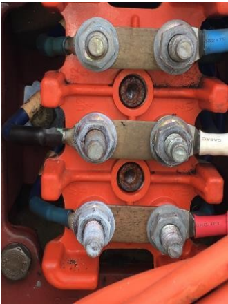
High Resistive crimp White Phase
