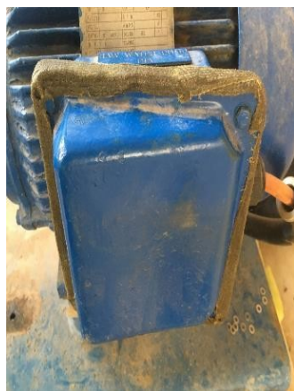
Denso Tape Waterproofing
