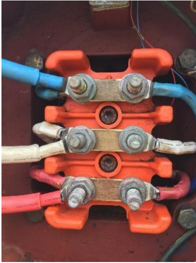
After relugging and connection
