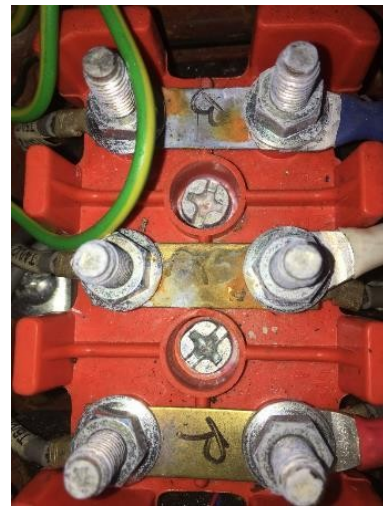
Moisture Ingress, Earth touching two phases
