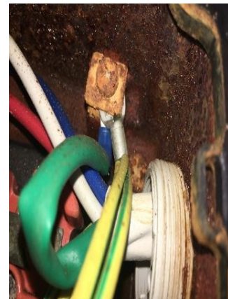
Moisture Ingress, Earth touching two phases
