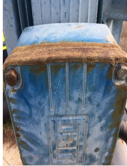
Denso Tape added to stop Moisture Ingress
