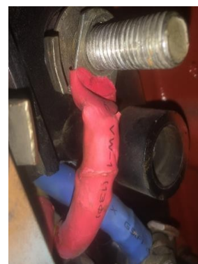
close to mounting bolt.VSD tripped
