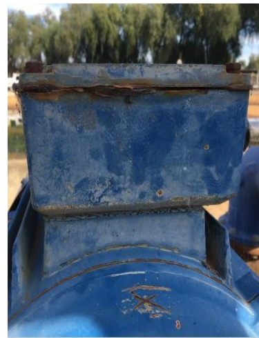
Terminal Box gasket failed
